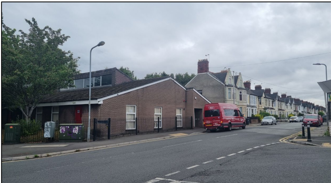
Figure 4: Existing Community Centre
